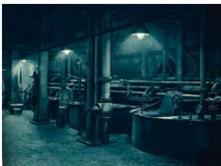
General lighting of a humidor with sealed KANDEM porcelain narrow angle light fittings, 1939.
