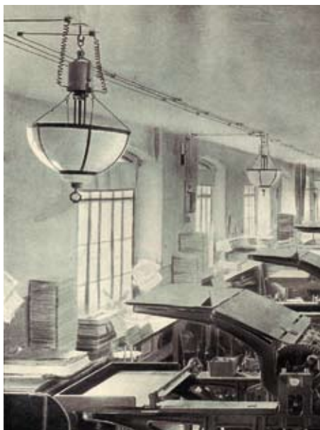
Steindrucksaal at the C. G. Röder Book and Note Printers, Leipzig with lights from KÖRTING & MATHIESEN, 1899.
