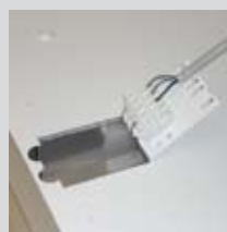
3 Insert the power supply cord into the clamp
